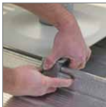
standing seam roof system installation
