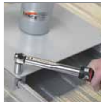
standing seam roof system installation
