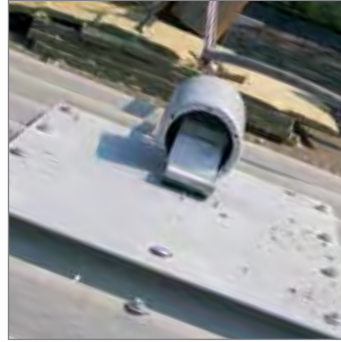
testing the system
